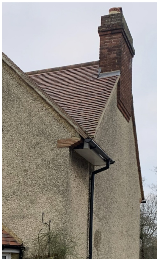
Figure 1: Soffits and corbels at present
