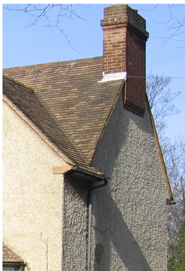
Figure 2: Soffits and corbels prior to loft conversion. The proposal will recreate this appearance
